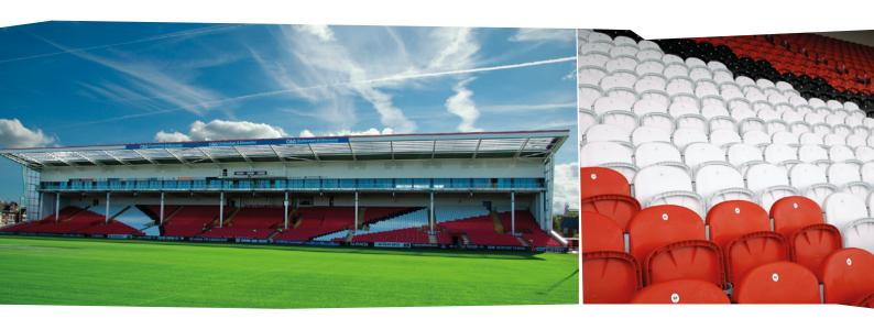
The design incorporated elevated hospitality boxes, located on a secondary balcony-level, high above the main spectator seating. This allowed a greater seating capacity in the main terraces; which consist of part-permanent and part demountable seating, with additional VIP areas.
