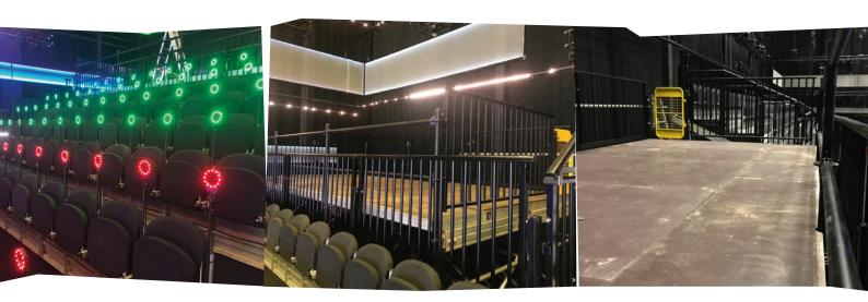
Production of the infrastructure was delivered in two stages, GL events UK's team erecting the tiered seating and platforms first, allowing the show's design team the floor space to create the set – staging, lighting, staircases, screens etc. Once this was in position, the team was then able to position the flat-floor seating. This was the same with the dismantle, again allowing the set to be taken down, and splitting the breakdown into two phases.
